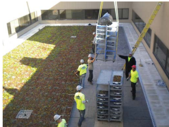
Live Roof tray system installation
