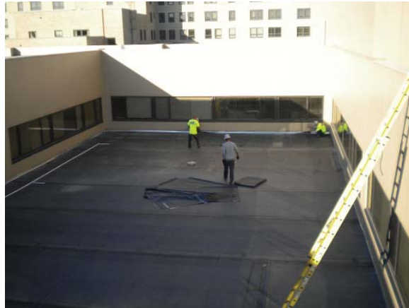
Roof area after tear-off
