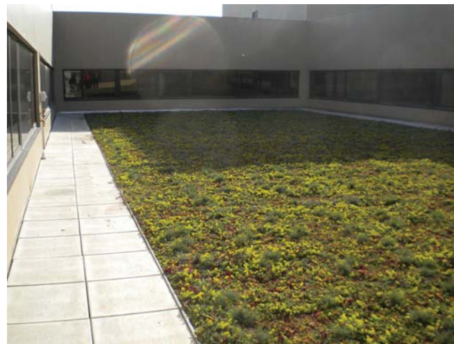
Overview of completed vegetated roof area
