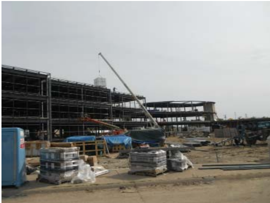
Preparing and placing materials
