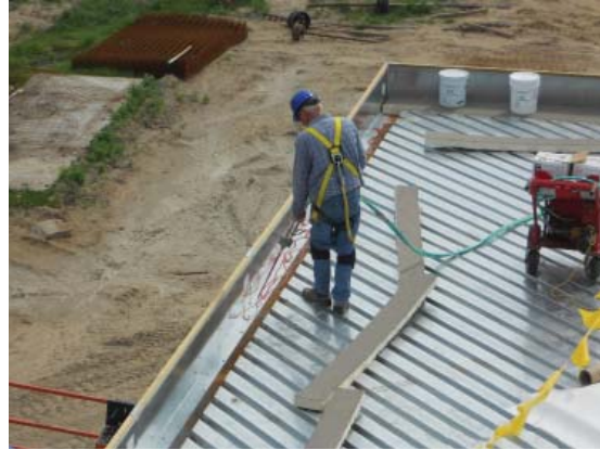
Insulation is being adhered with VOC free adhesive
