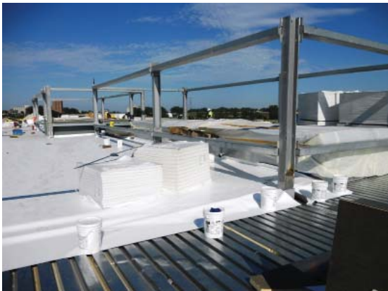
Roof at RTU screen wall.
