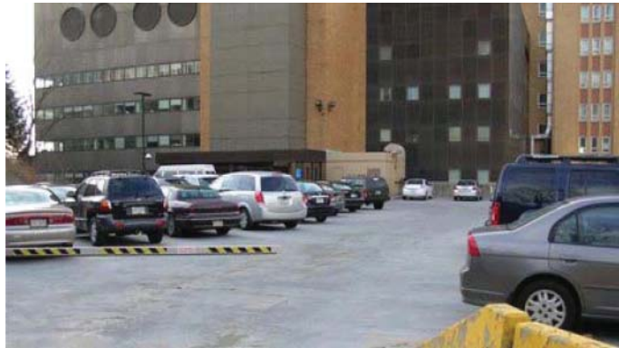
Partial overview of level 5 of the parking structure
