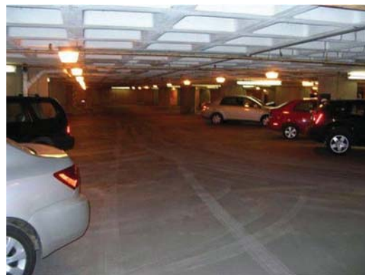
Overview of Western Psychiatric Institute & Clinic parking structure level 2
