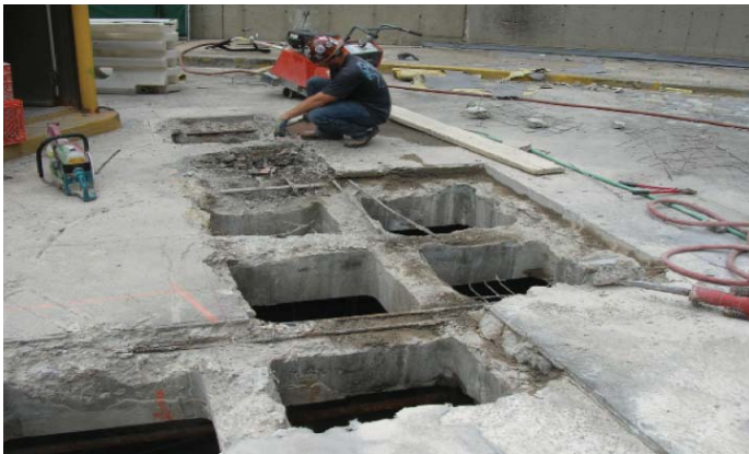
Western Psychiatric Institute & Clinic parking structure construction
