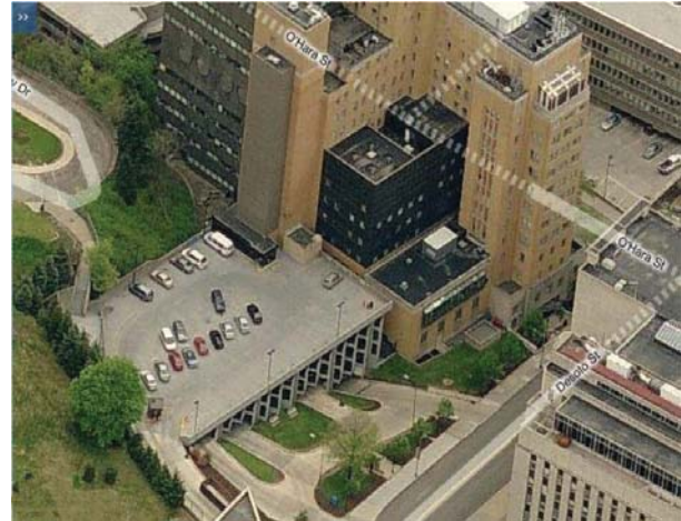
Overview of University of Pittsburgh Medical Center - Western Psychiatric Institute & Clinic parking deck
