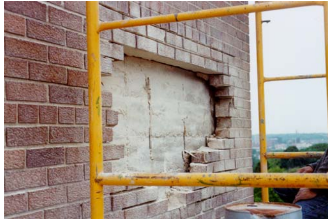
Demolition included removing degraded masonry units and ties.
