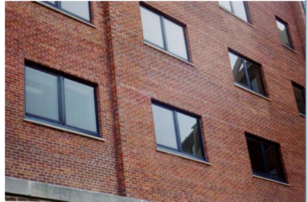
Overview of completed wall restoration.
