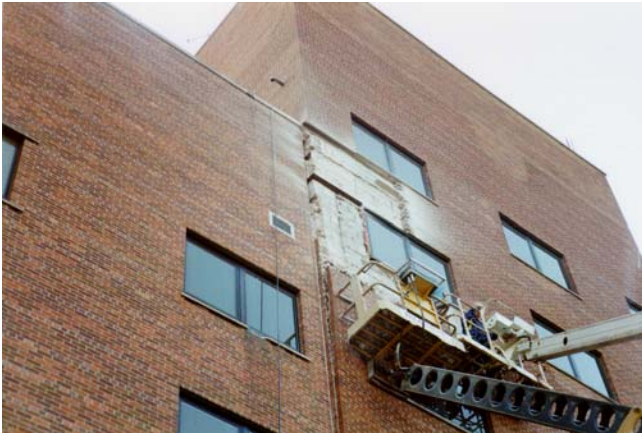
Overview of work in progress.
